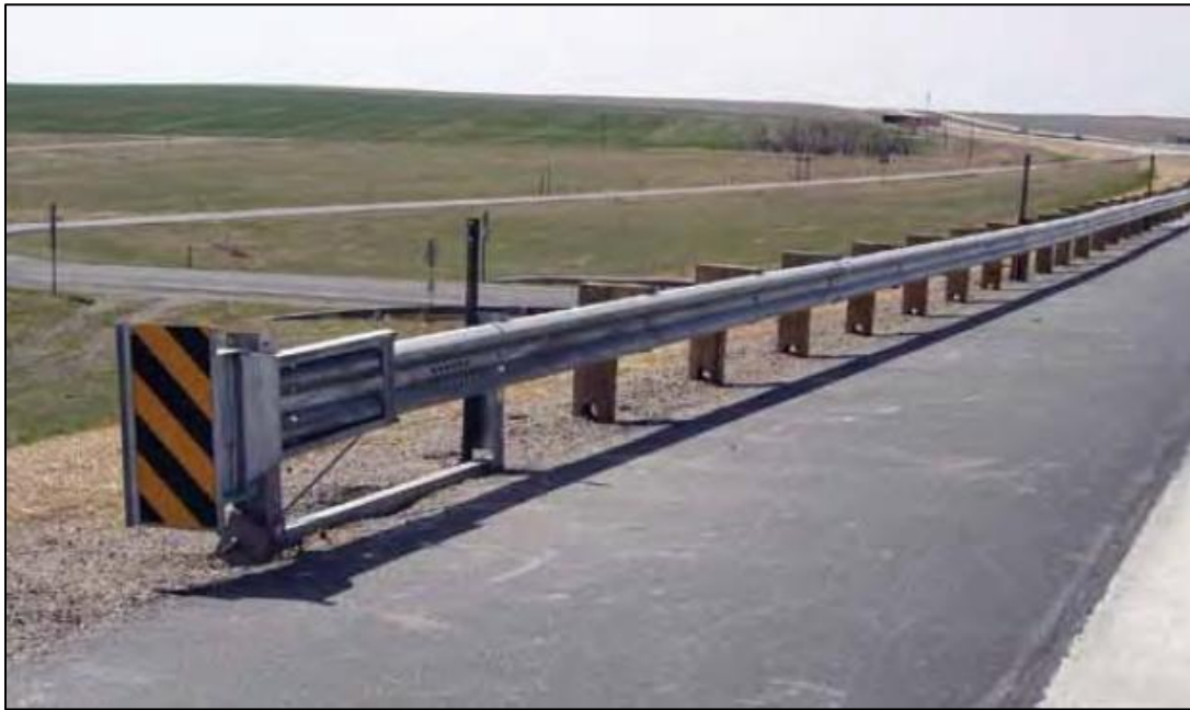
Sample guard rail end treatment and posts (Source: AASHTO Roadside Design Guide 4 th Edition)
