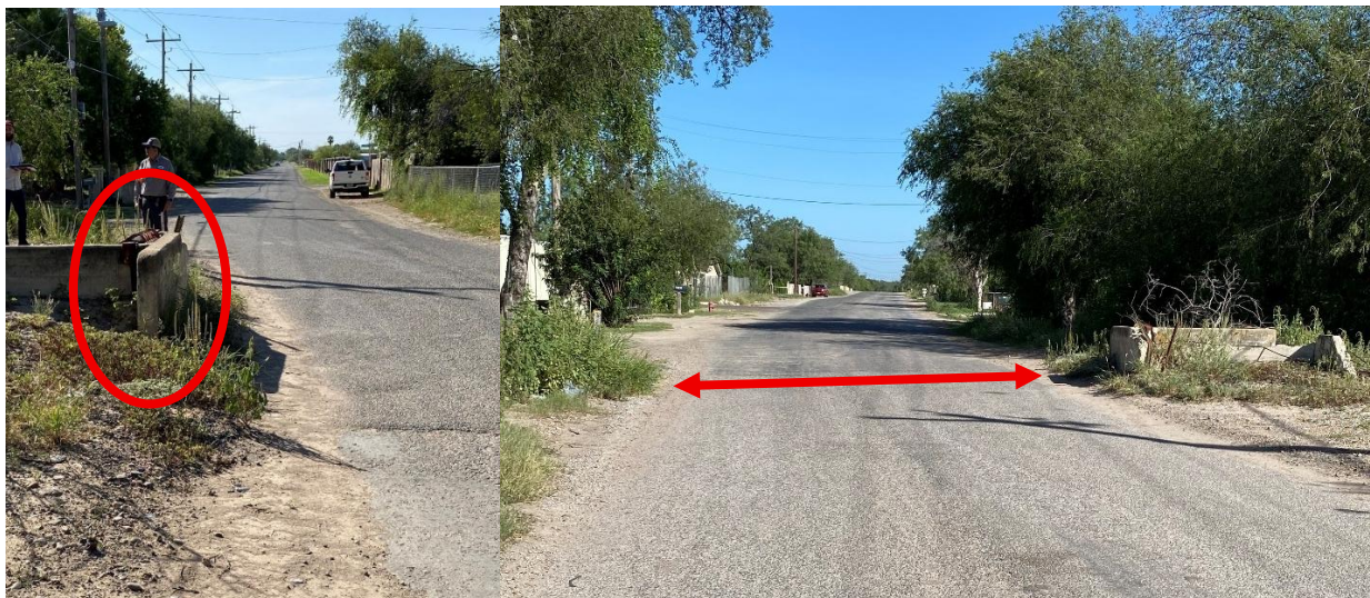
Unprotected headwalls at narrow passage on Rosita Valley Road (Source: FHWA)
